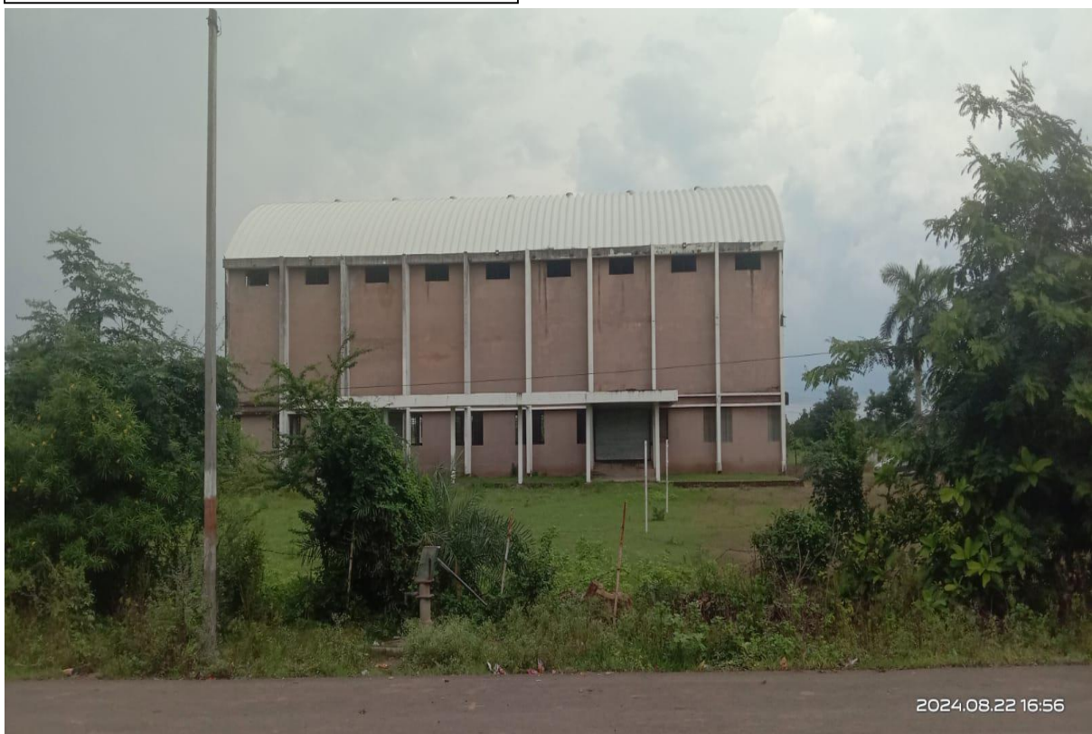
Wind driven roof of college indoor stadium
