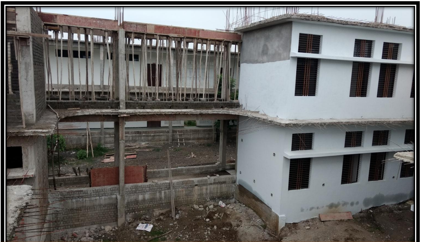
Construction of Class Rooms and Laboratories
