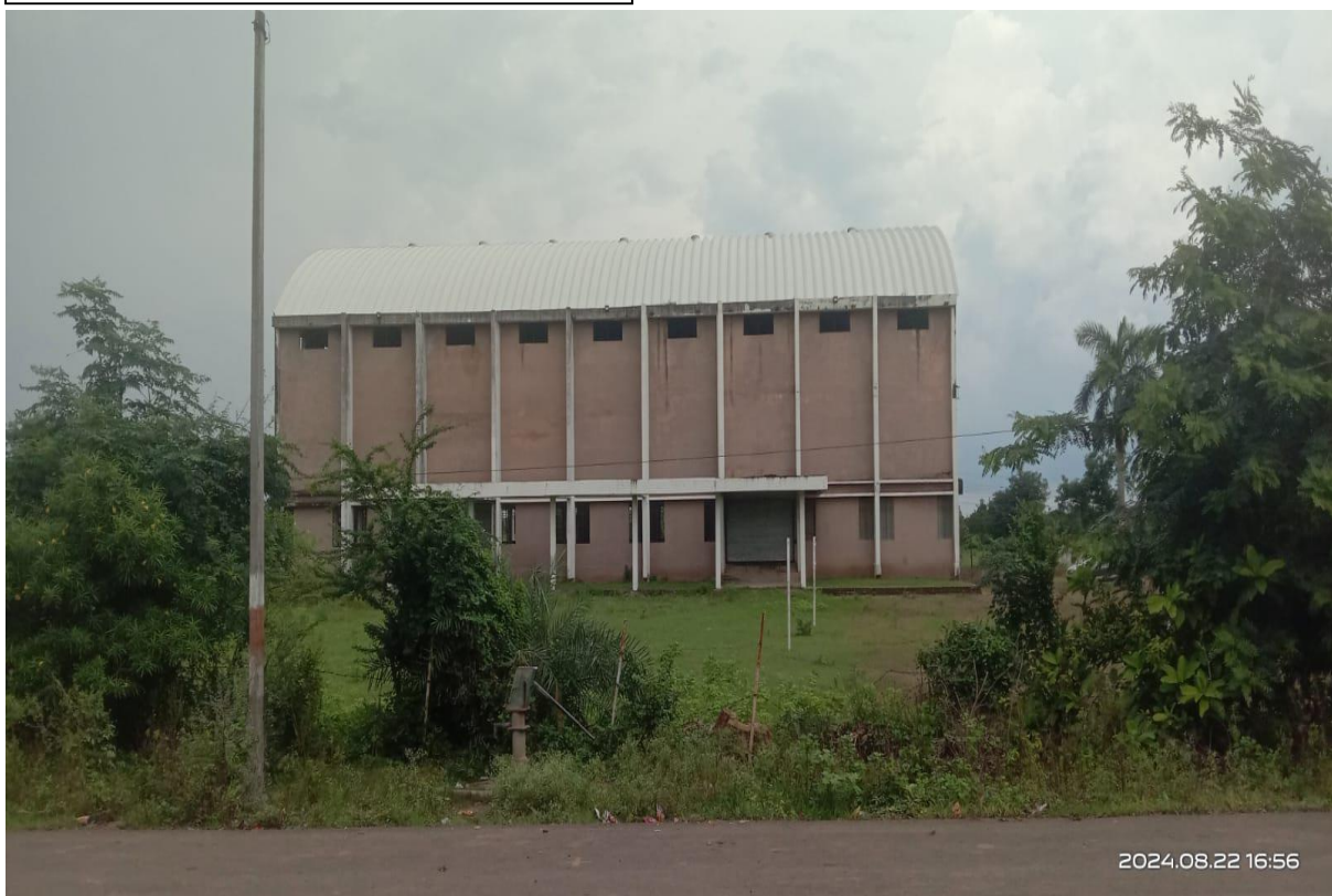
Wind driven roof of college indoor stadium
